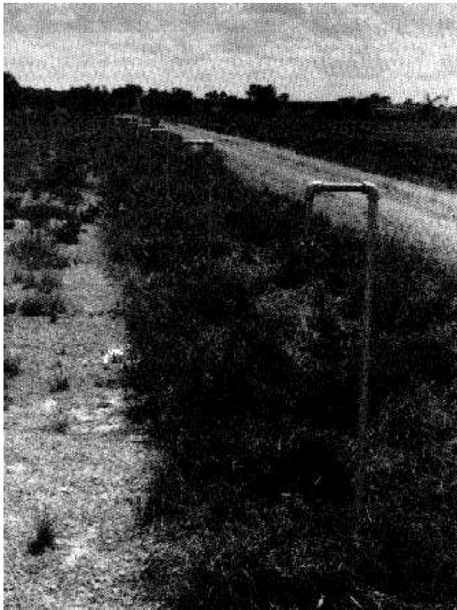
FIGURE 6-3 DISTRIBUTION FOR OF USING LOW PRESSURE FAN SPRAY NOZZLES
