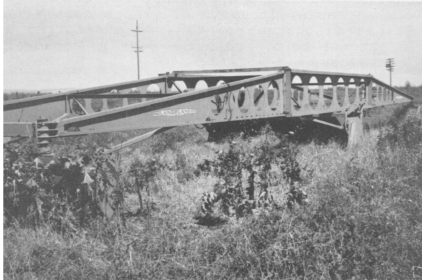
FIGURE 6-5 LAND PLANE USED FOR FINAL GRADING
